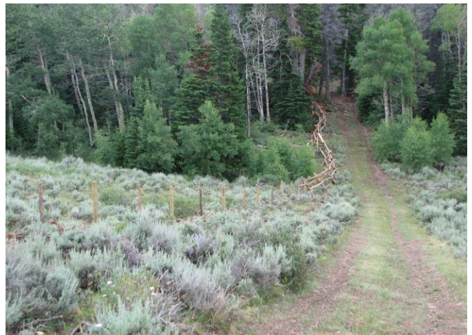
The Miller Mountain cross fence consists of buck and pole and 3-wire lay down fences.
